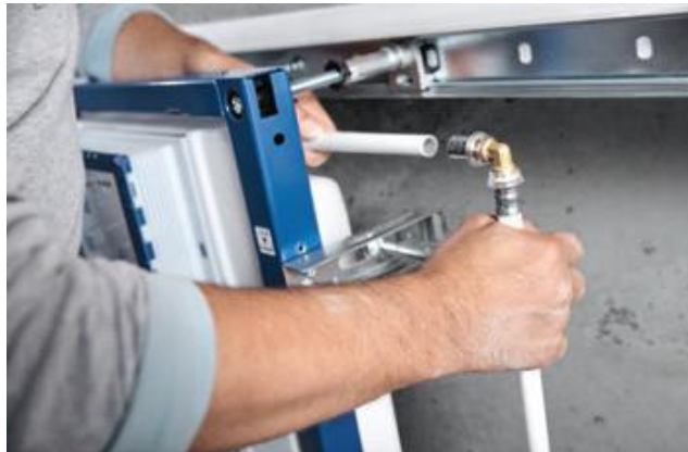
↑ Inserting the brass fitting into the pipe does not require special efforts.
