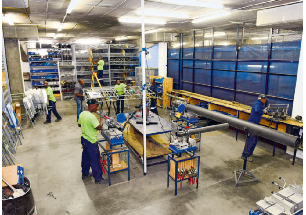
↑ Geberit HDPE pipes being butt-welded at the nearby workshop: the company Modern Plumbing Works was able to meet the ambitious schedule thanks to prefabrication.
