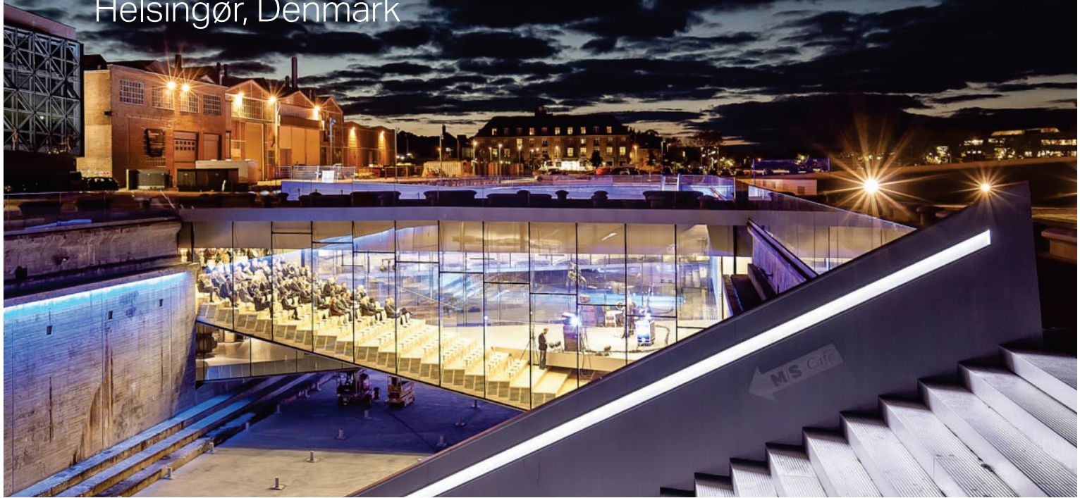
↑ As part of the museum construction process, the old dock wall was completely uncovered and the dry dock left empty.
