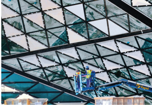
↑ Putting the finishing touches to the conference center.
