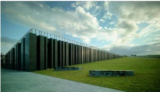
Local stonemasons delivered a total of 186 columns made of black basalt. The stone was quarried near the Giant's Causeway.
