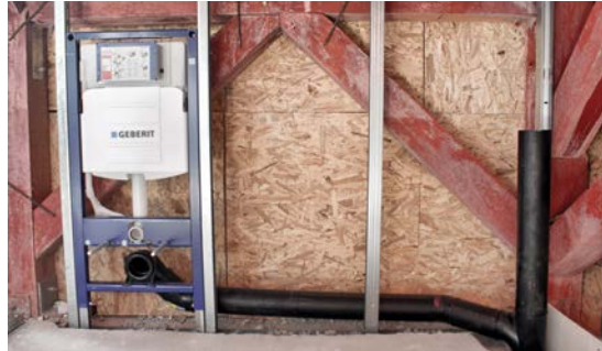
Whether commercial clerks, mechanics or plastics technicians – Geberit apprentices show their plumbing skills during the social project in Romania.
