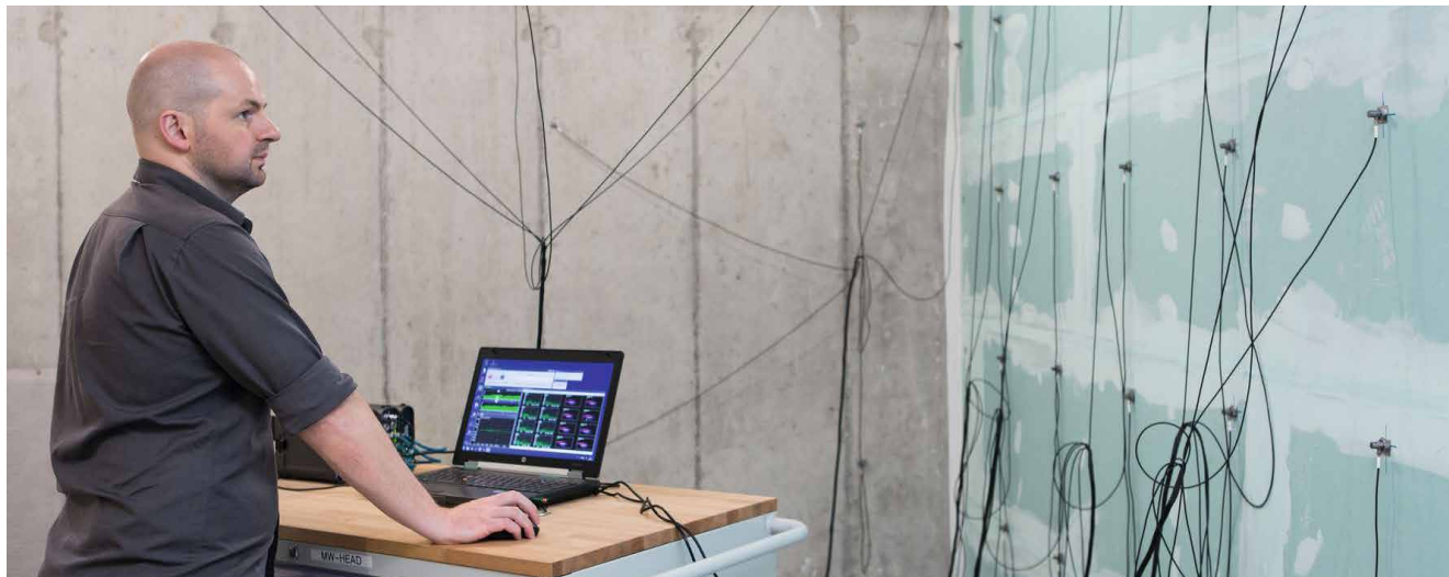
Samuel Pasteur, acoustics specialist at Geberit, measures the sound transmitted from a concealed installation to a neighbouring room using acceleration sensors.
